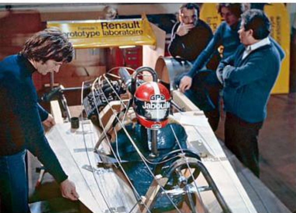
Hubert, de Cortanze, Guénard. By now they were beginning to put templates on the wooden mock-up to create the shape of the body. Parts of the A500 were used to create the design, as can be seen from the yellow-painted rear wing unit.
